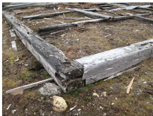
Figure 2. Wood in soil contact is decayed by both soft-rot and brown-rot fungi.
