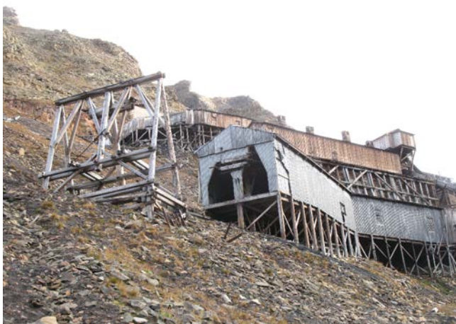
Figure 1. On Svalbard there are many wooden constructions left from earlier industrial activity.
