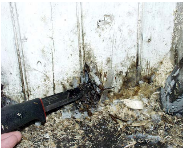
Figure 6. Typical growth conditions for Leucogyrophana mollis in lower part of walls, close to soil.
